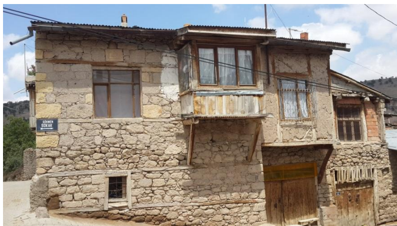
Figure 19. On the facade of a house, stone wall with fitches and the wooden exedra overflowing toward the street on beams and bolstered with buttresses is seen.
