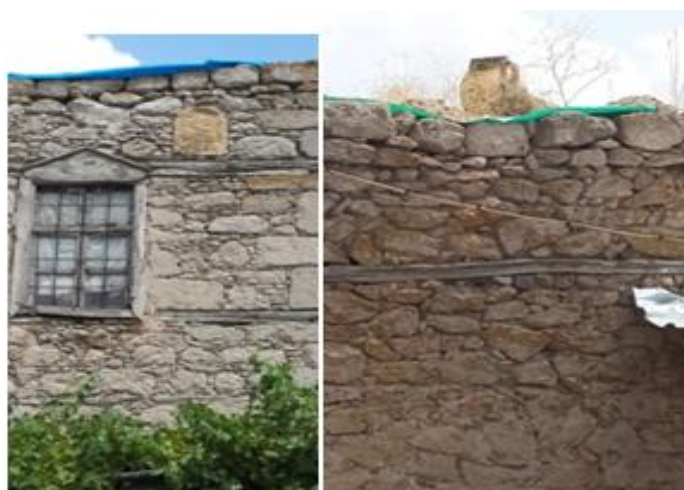
Figure 21. Yellow Epitaph Stone on the Facade of the Ayyıldız's House
